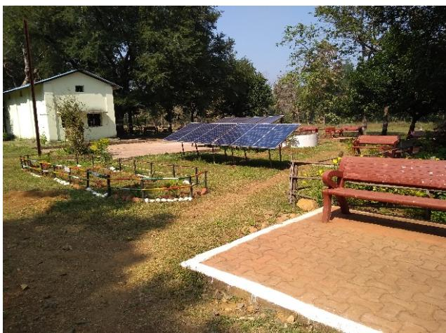
Solar Panels -Only source of electricity – used to run 2HP pump
